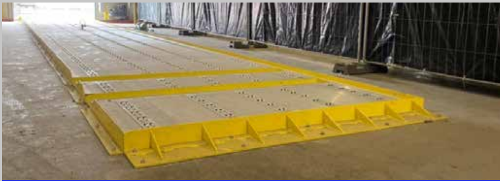
FORKLIFT PROTECTION STRIPS
